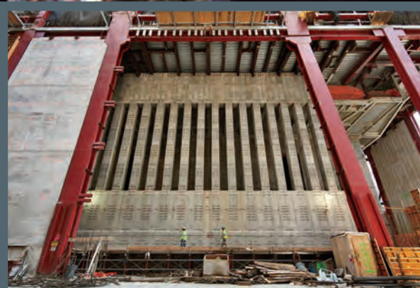
One World Trade Center's 186-foot-high base is made of the strongest concrete ever used in New York City architecture.
