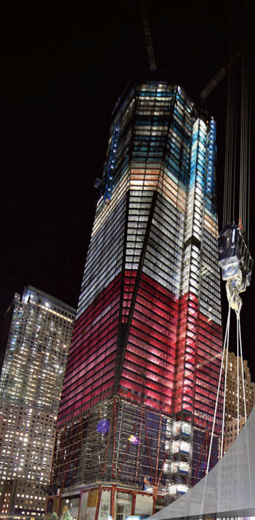
One World Trade Center's 186-foot-high base is made of the strongest concrete ever used in New York City architecture.
